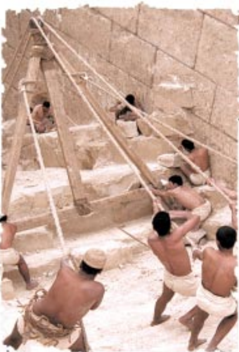
The laborers haul stone blocks into the King's burial chamber using an A-frame and ropes.
