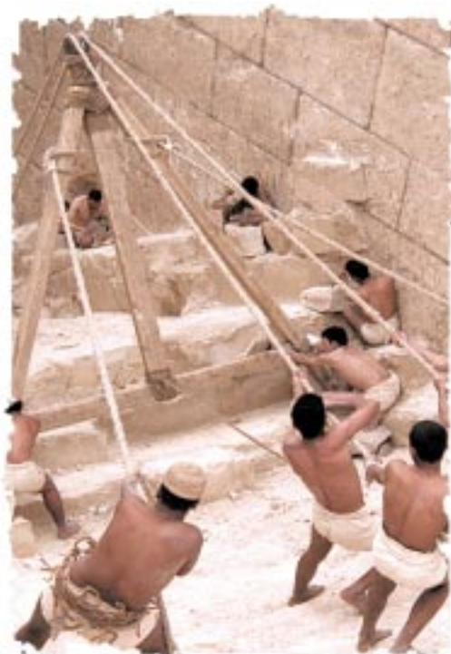
The laborers haul stone blocks into the King's burial chamber using an A-frame and ropes.
