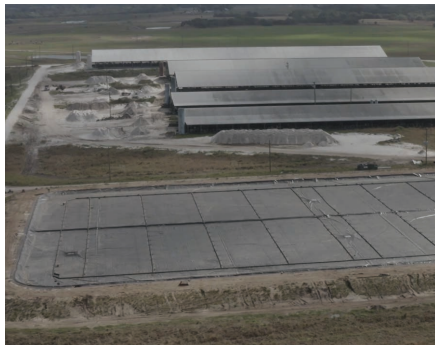
Larson Dairies in Okeechobee, Fla., use anaerobic digesters to convert methane, a greenhouse gas released from cow manure, into a source of electricity.
